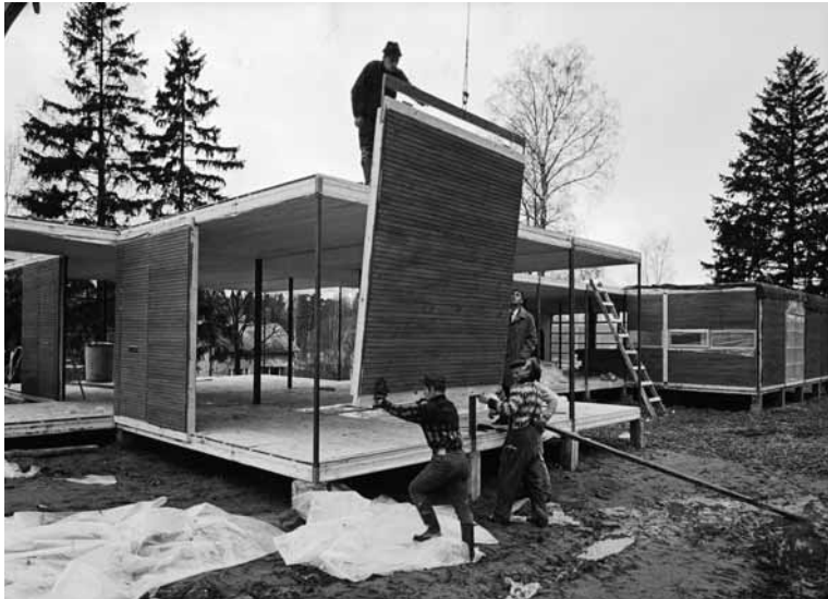
Domino element housing system under construction, 1968.
