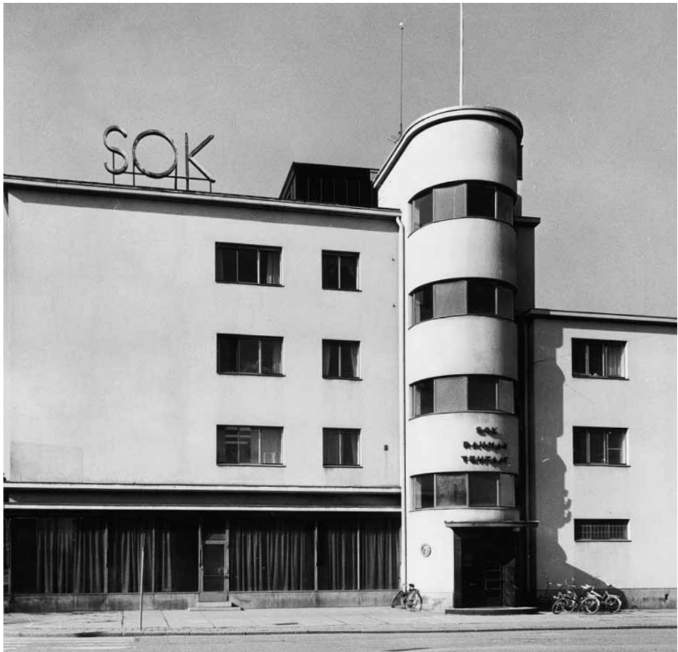
Erkki Huttunen, SOK Office Building, Rauma, 1930–31.
