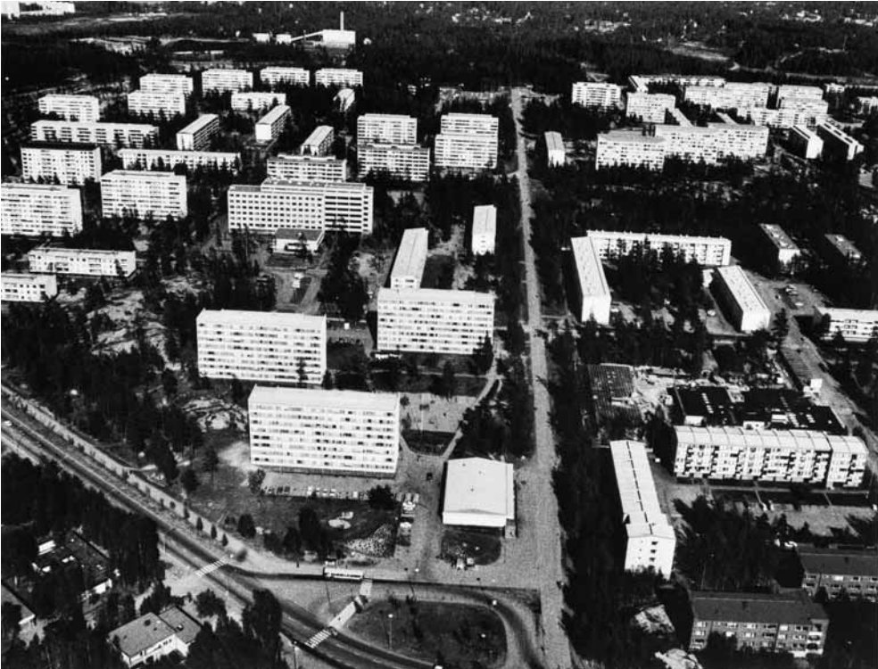
Myllypuro, Helsinki, an example of rectilinear prefabricated housing from the 1970s.
