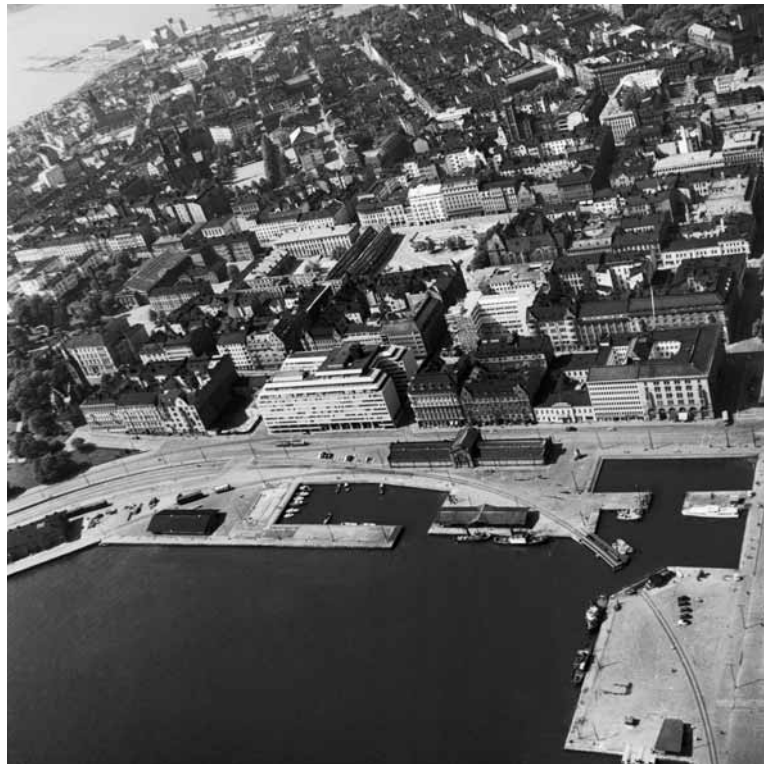
Viljo Revell and Keijo Petäjä, Palace Hotel and Centre for Industry, Helsinki, 1952.
